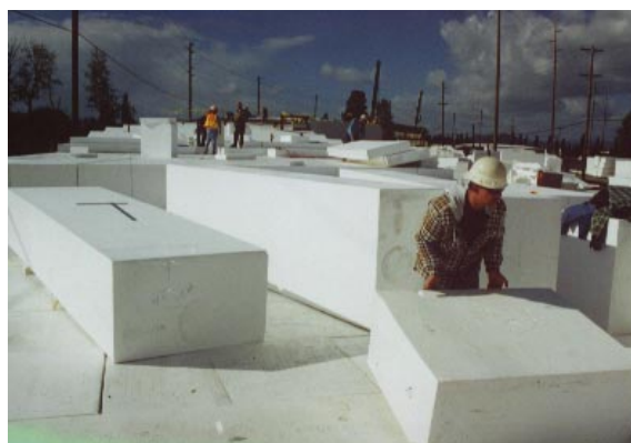
An Ostrander Rock & Construction worker moves Geofoam blocks into place. Each 16 foot-long block weighs approximately 280 pounds.
