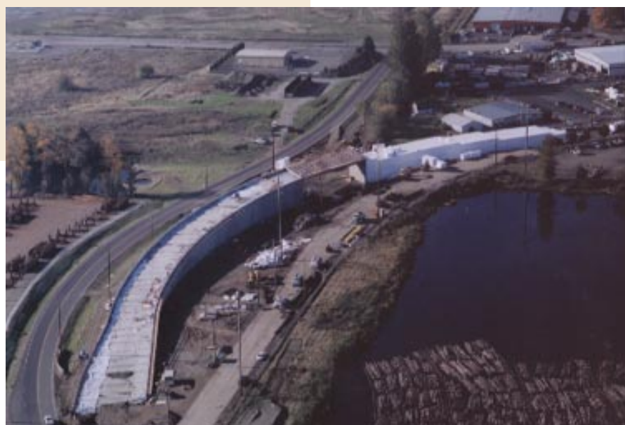
Fibre Way Grade Separation project under construction in November 2001. Geofoam fill can be seen at the top right.
