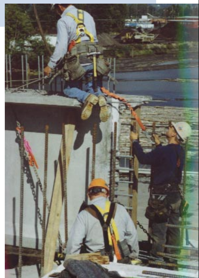
Five Rivers Construction workers steady the first of seven pre-cast concrete girders as they are moved into place atop the Fibre Way Grade Separation project.
