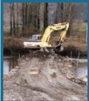
Filling in a log pond for the Industrial Rail Corridor.
