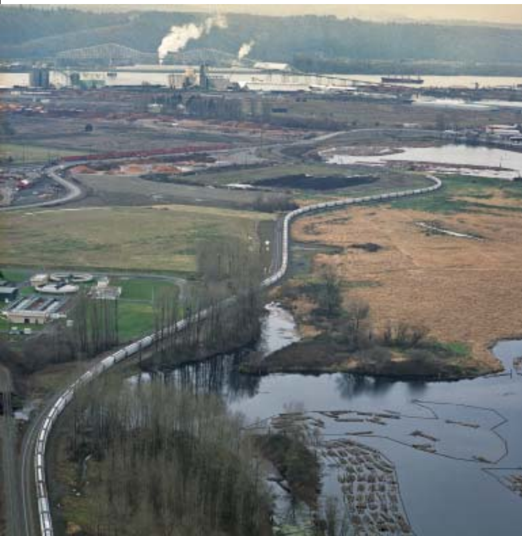
The first train on the new rail corridor can be seen winding towards the Port's Marine Terminal Complex in this January 2005 aerial. Trains can now carry more rail cars to the Port without encountering road crossings.
