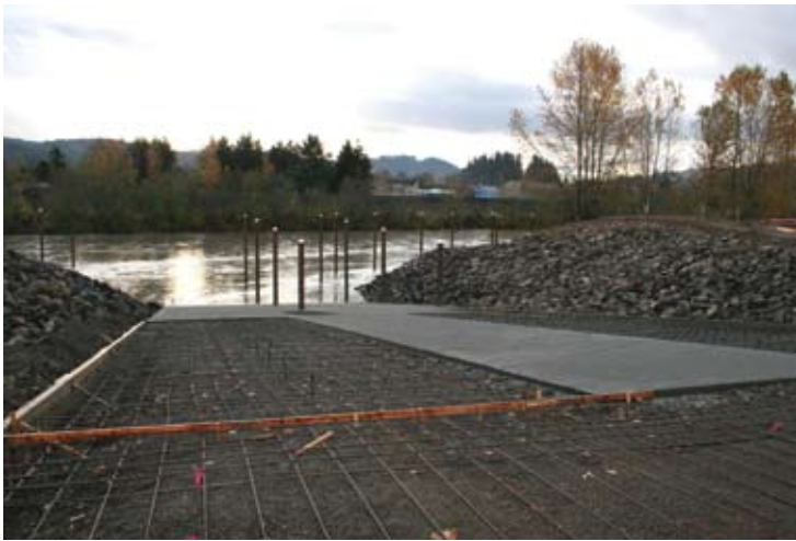
Crews continue to work diligently on the Castle Rock Boat Launch
